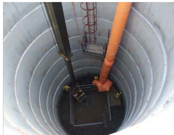
Excavation of Drop Shaft A for TBM Retrieval
