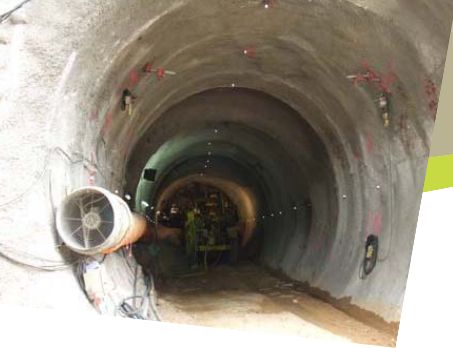
Branch Tunnel Chamber Constructed in Softground
