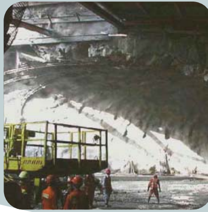
Construction of the HKC Tunnel using Drill and Blast Techniques
