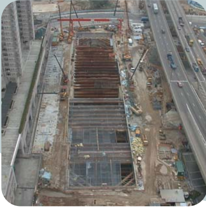
TBM Launch Chamber, Tsuen Wan
