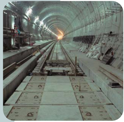
Completed Tsing Tsuen Tunnel
