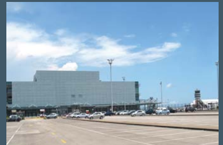
Macau International Airport Sustainability Plan and LEED EB-OM Certification
